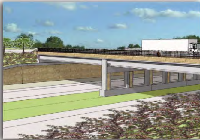
159th St. Bridge over US 69 Looking Southeast
